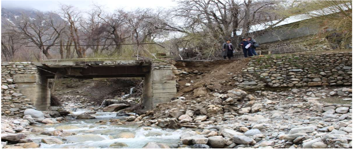
Current condition of Bridge No.5, Tekharv jamoat
