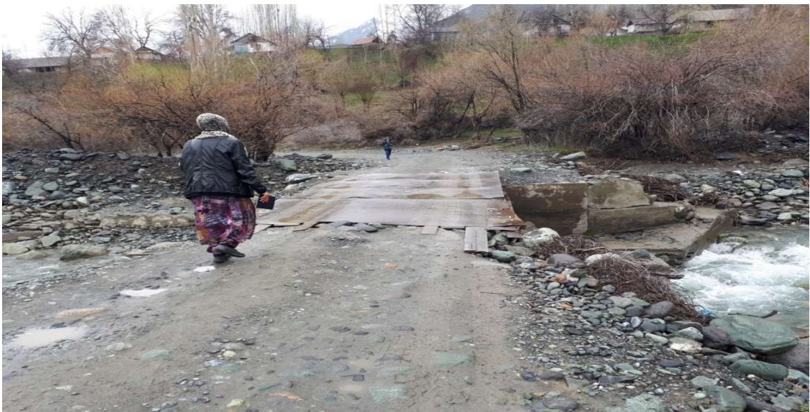
Current condition of Bridge No.4, Tekharv jamoat
