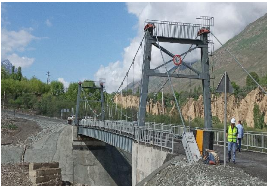
Bridge No. 7, Vanj district
