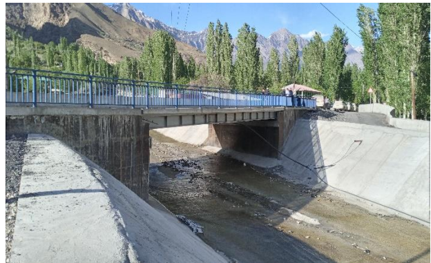
Bridge No. 9, Rushansky district
