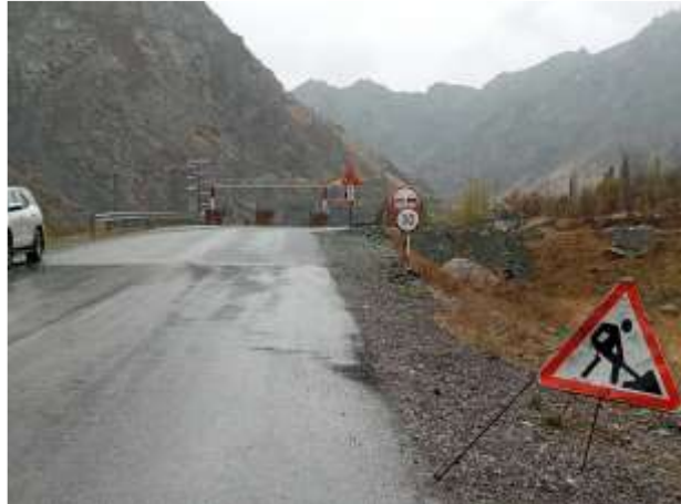
Bridge No. 14. Road signs
