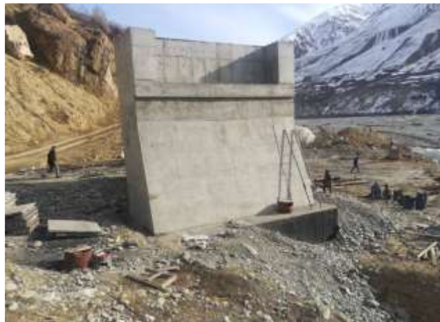
Bridge No.6. Completed support
