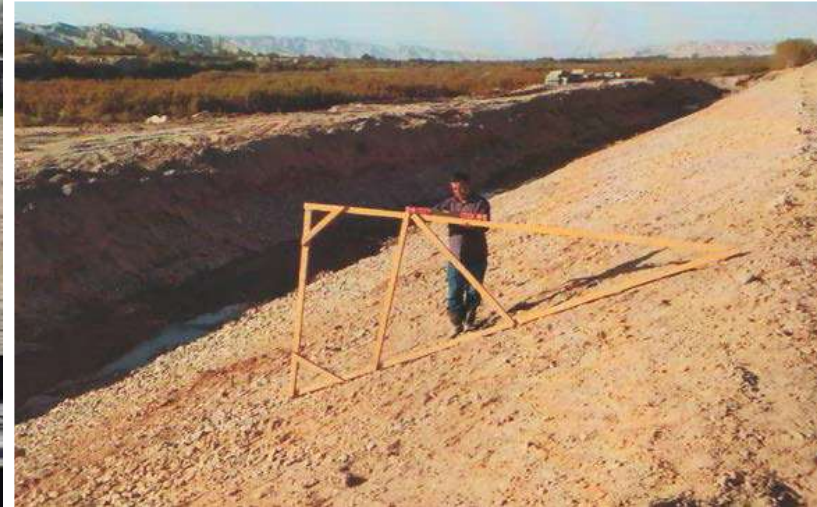
Kabadiyan. Preparing slopes
