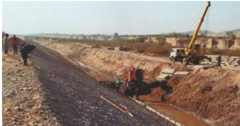
Kabadiyan. Fastening the apron
