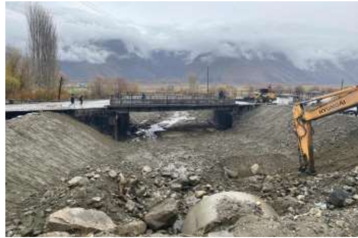
Bridge No.9. Strengthening the slop
