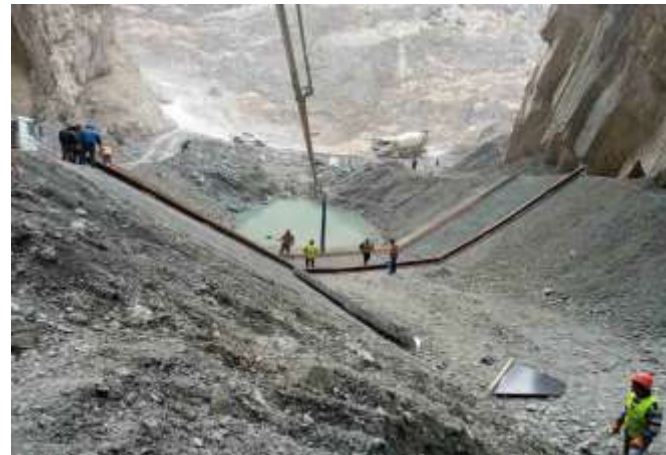
Bridge No.15. Strengthening the upper channel
