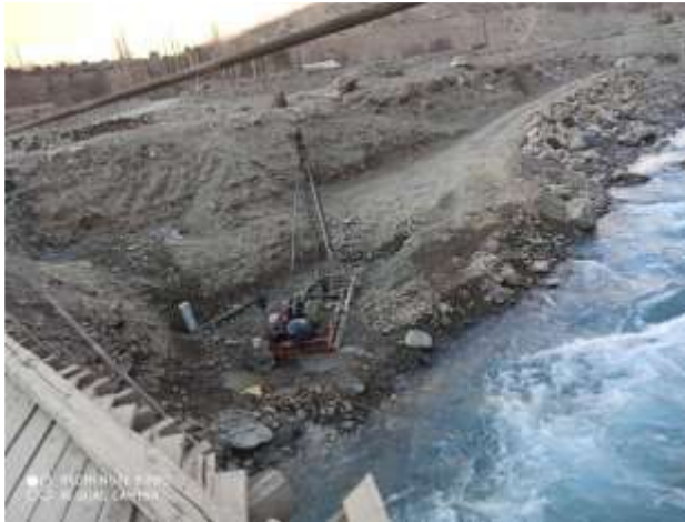
Bridge No.3. Bored works
