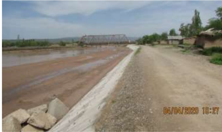
Vose. Dam restoration. Surkhob river.
