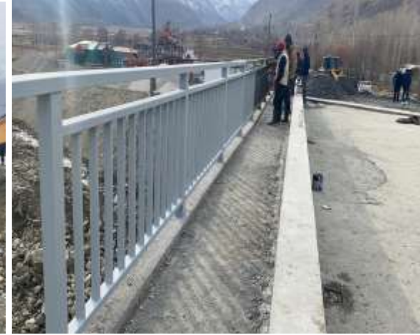
Bridge No.9.Okraska bridge railing
