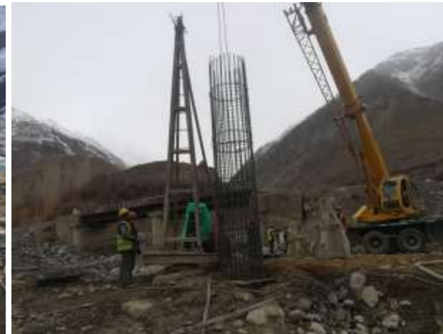
Bridge No. 7. Pile concreting
