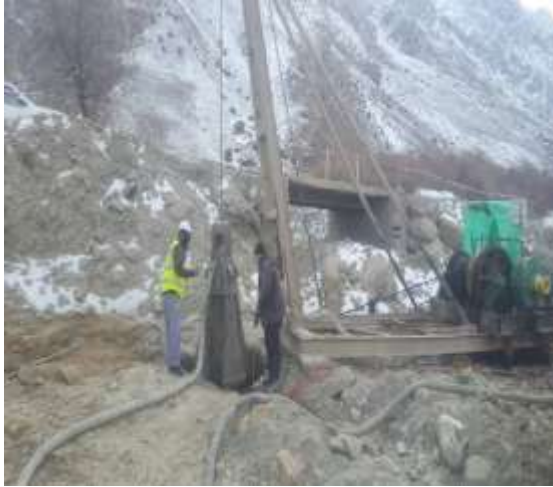
Bridge No. 8. Bored works
