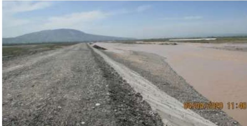
Vose. Yakhsu river. Rebuilt dam. Larhobi.
