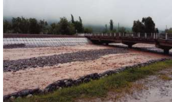
Kulyab. Rebuilt dam. Zarkala site
