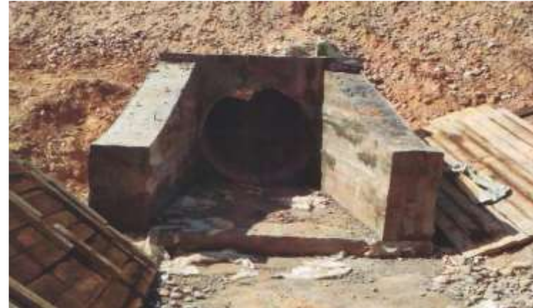
Kabadiyan. Construction of a pipe crossing
