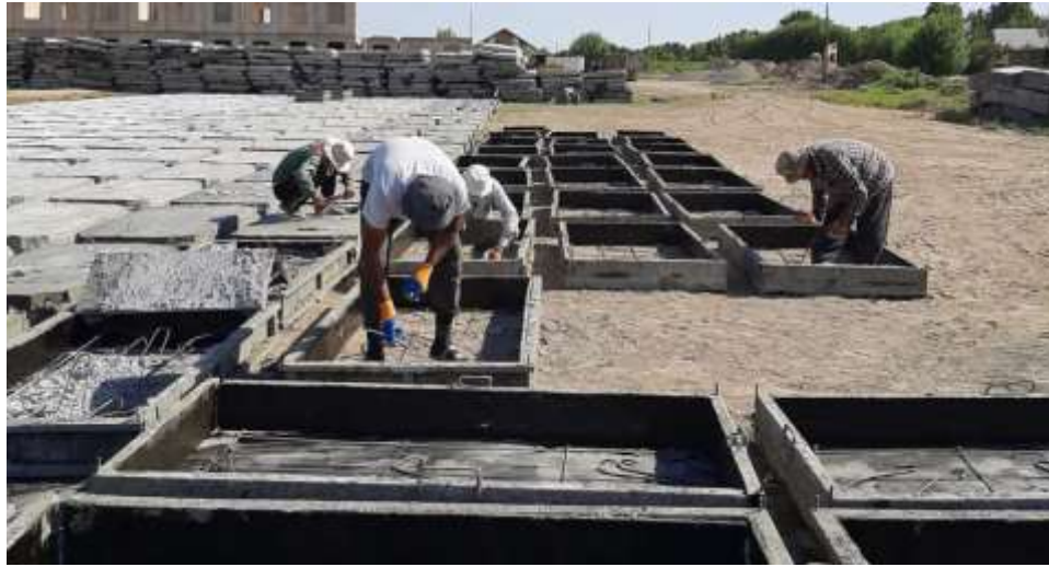
Kabadiyan. The process of making reinforced concrete slabs.
