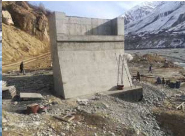
Bridge No.6. Completed support
