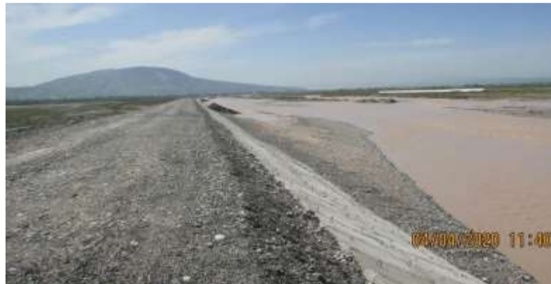
Vose. Yakhsu river. Rebuilt dam. Larhobi.
