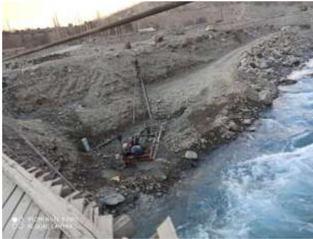
Bridge No.3. Bored works
