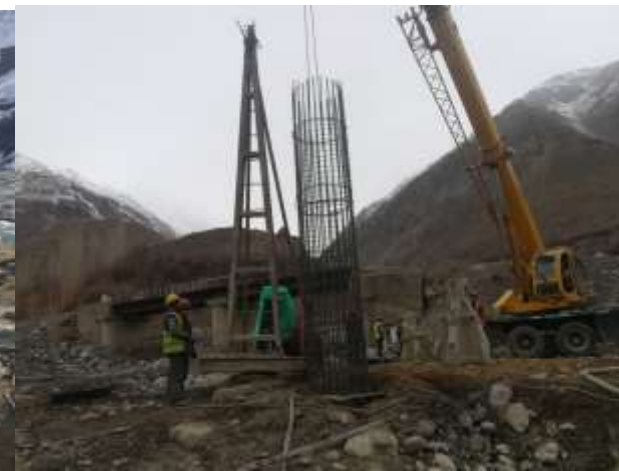
Bridge No. 7. Pile concreting
