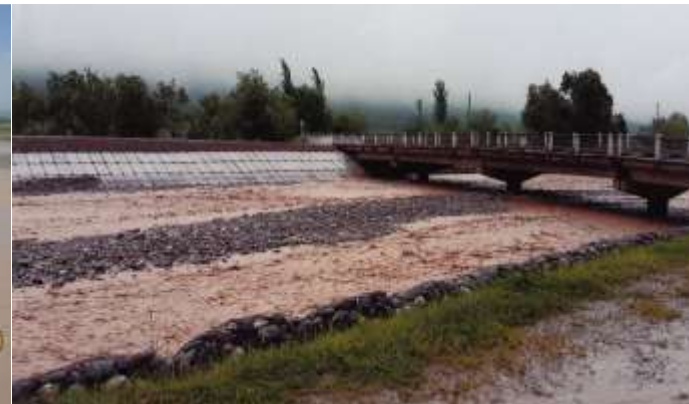
Kulyab. Rebuilt dam. Zarkala site
