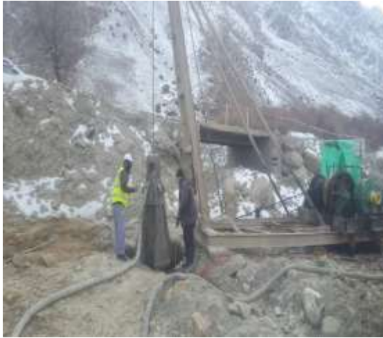
Bridge No. 8. Bored works
