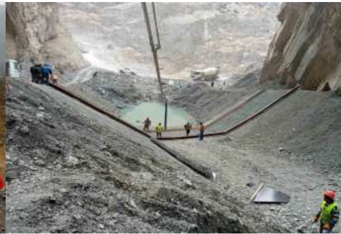
Bridge No.15. Strengthening the upper channel
