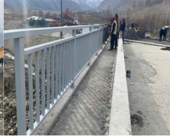
Bridge No.9.Okraska bridge railing
