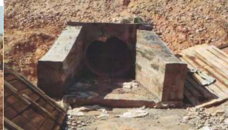
Kabadiyan. Construction of a pipe crossing
