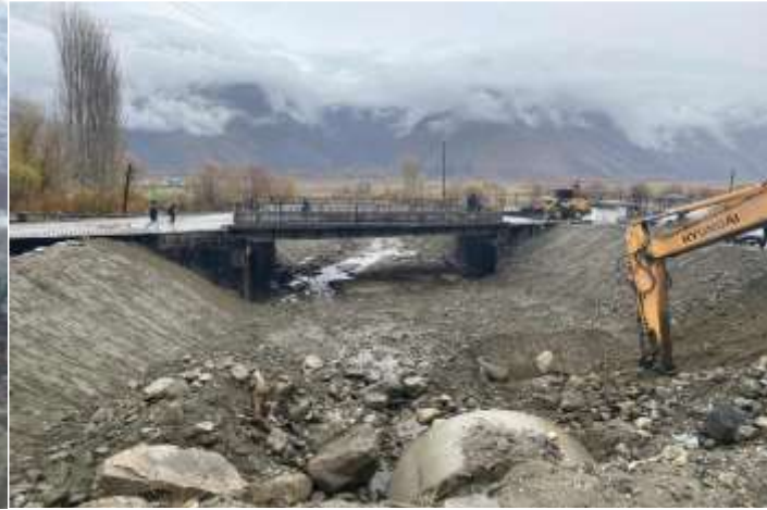
Bridge No.9. Strengthening the slop
