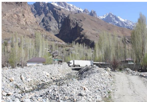
Bridge No. 9 before rehabilitation
