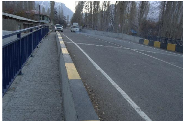
Bridge No. 9 after rehabilitation
